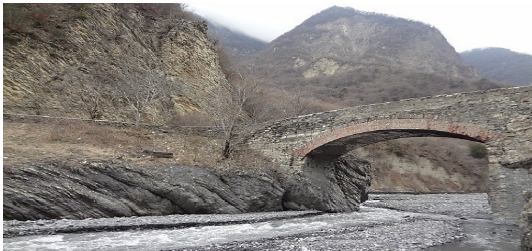
Figure 9. Southern slope of the Greater Caucasus, Ilisu Bridge, and alluvial fans of the Kurmukchay River, Gakh District, Azerbaijan
